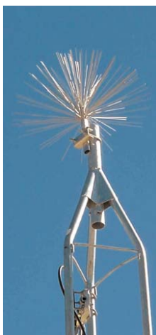
Multiple points can dissipate larger charges.
